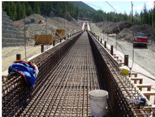
2008 Olympic bobsled run in Vancouver under construction.
